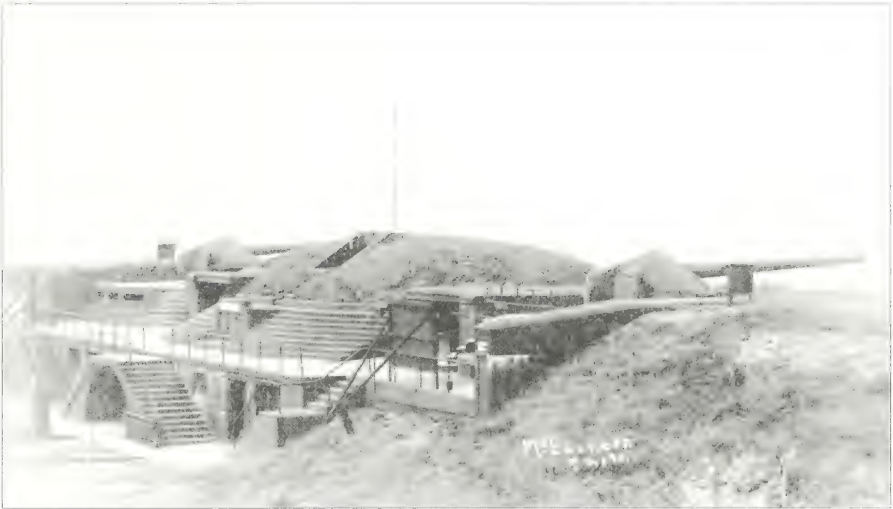
Figure 2.81. Open battery commander's station at Battery Peck, circa 1905–10. Prior to the modifications in 1920, the battery commander for Battery Peck stood on an open, concrete platform centered between the two emplacements (Thomas Hoffman, Fort Hancock , Charleston, SC: Arcadia Publishing, 2007).
